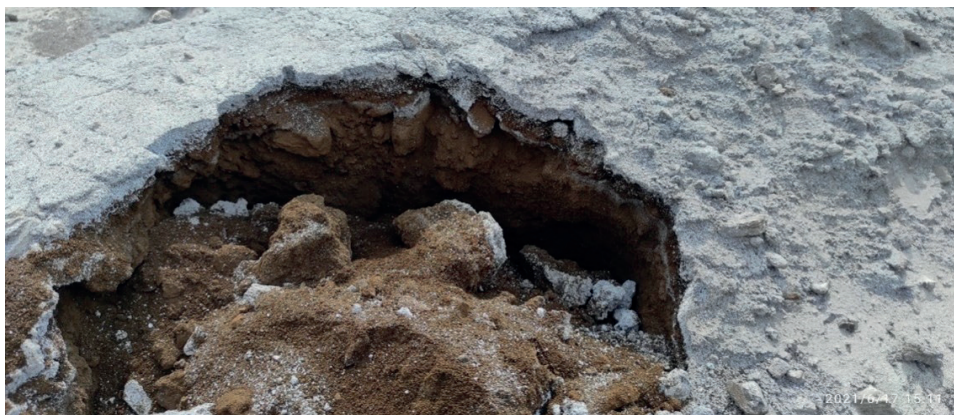
Figure 2. View of upper and lower layers of bauxite sludge on sludge storages of Pavlodar aluminum plant
