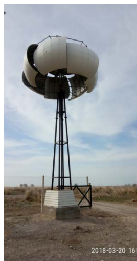
Figure 1 – “Torus” Wind Power Plant
